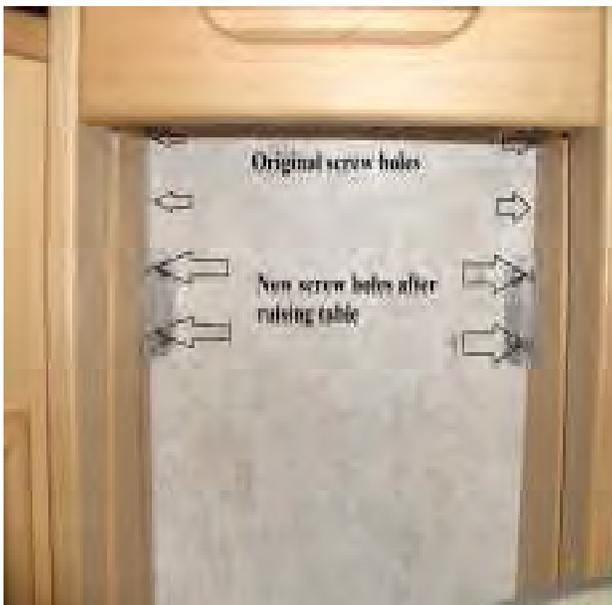
Now remove the 4 screws in the cross braces as seen in the photo. The cross braces stay attached to the frame.
