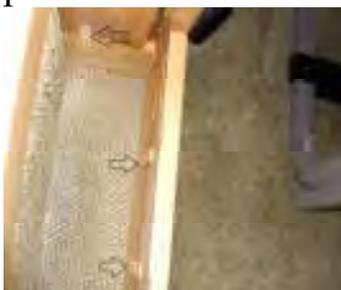
You need to notch the riser to fit the wall just like the original base.
